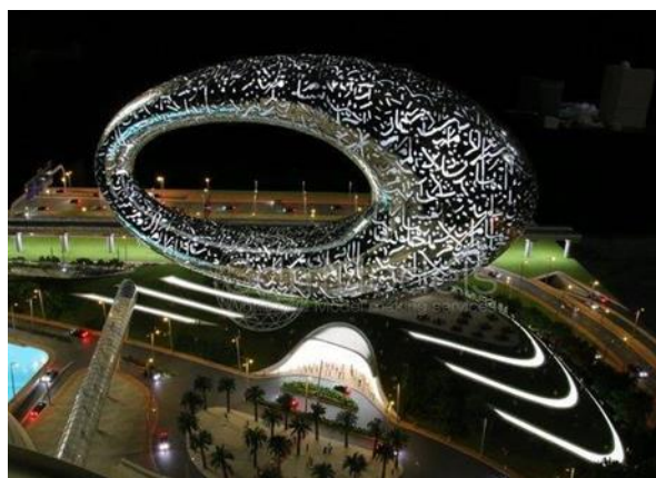
Shape 21- night image for the future museum shows the cladding as a source of lighting for the building.
