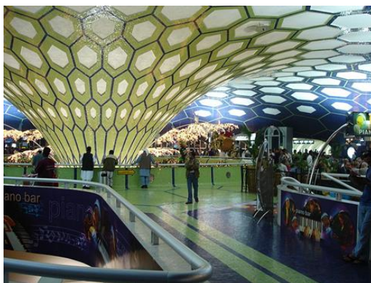
shape 24 shows the ceramic claddings and the Islamic geometrical units.
