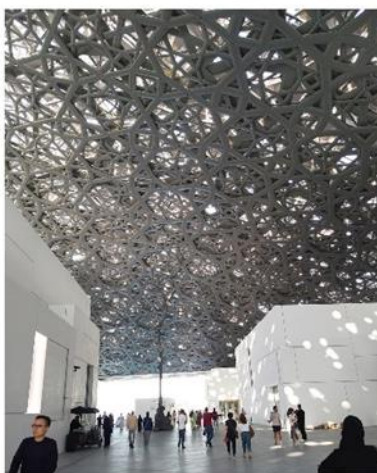
Shape 23 the image on top shows the external shape of the doom- the lower image shows the shape of the internal dome.
